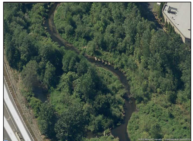
Completed Phase I project upstream
