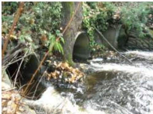
Pre-project: fish passage barrier culverts
