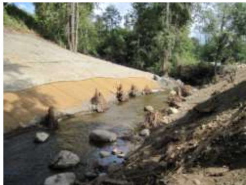
Post-project fish passage barrier culverts removed and stream restored
