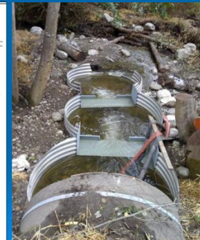
Completed Project: October 19, 2010
