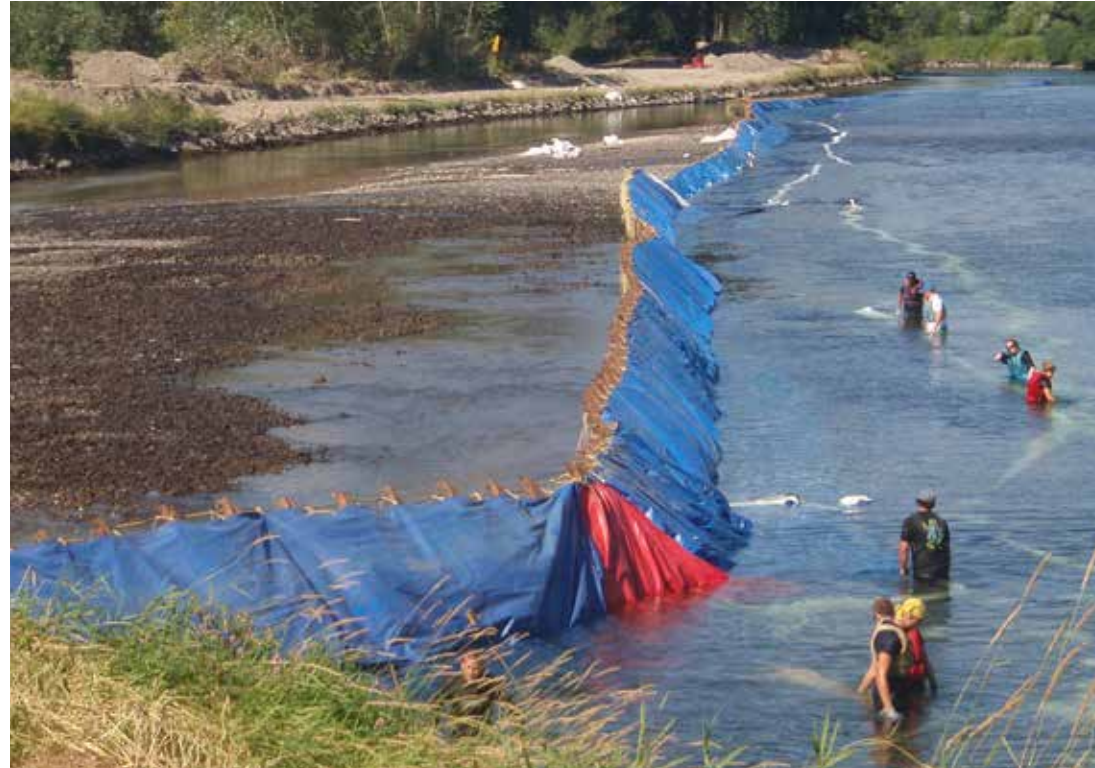
A temporary dam protects water quality during construction of the Chinook Bend project.
