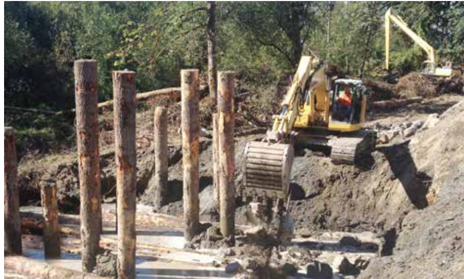
Pile-supported structures built at the Upper Carlson site provide flood protection as the river migrates.
