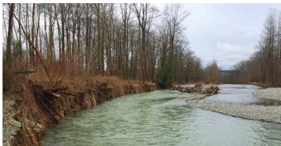
Tolt River after levee removal in 2015
