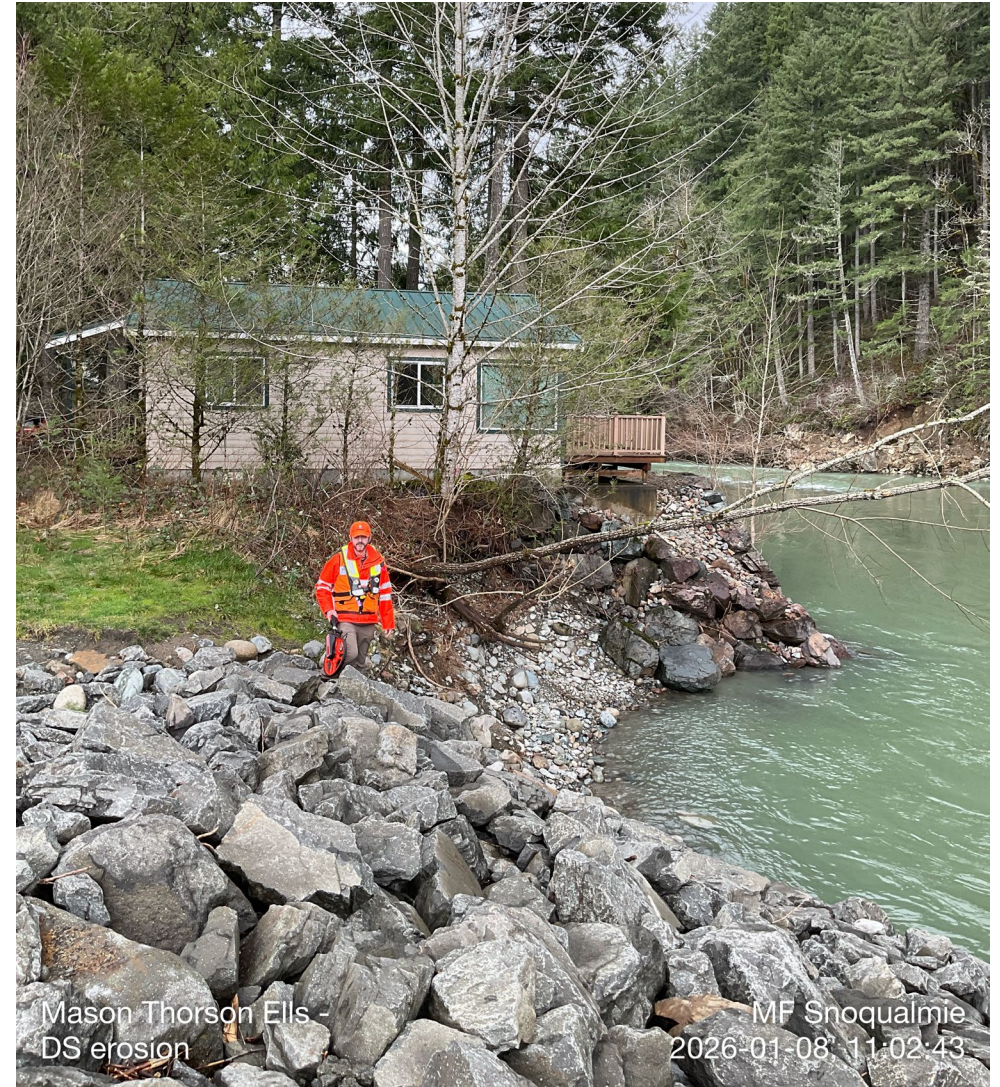
King County geologist inspecting damage on the Middle Fork Snoqualmie River, Jan. 8, 2026
