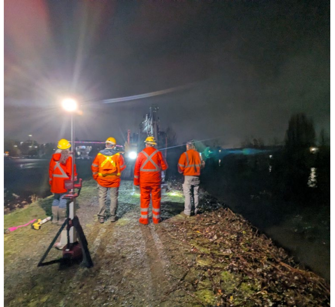
Roads Special Operations Crew, Green River, Dec. 23, 2025
