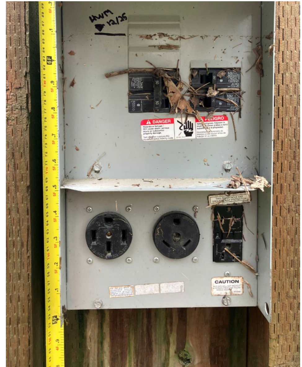
High-Water Mark: Seed Line at Tolt-MacDonald Park
