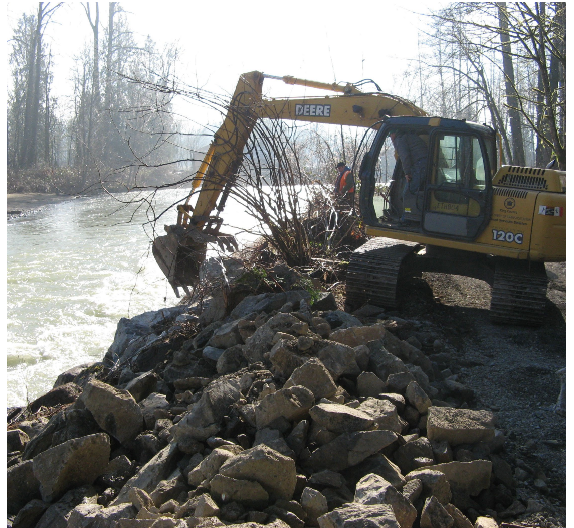
2009 emergency repair along existing Lower Frew levee
