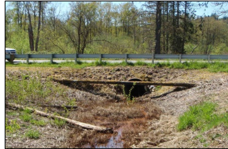
Existing culvert under SR 203
