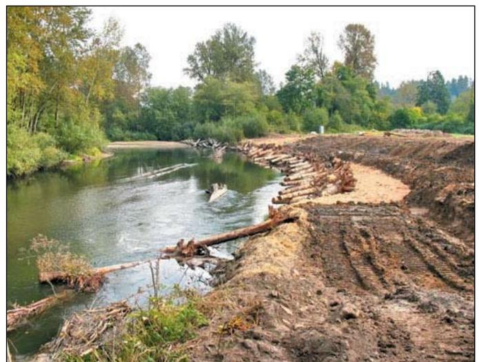
*The Fenster restoration in Auburn under construction in October 2008, showing large wood used to armor the toe of the bank while providing shelter for fish. Photo courtesy of King County.*
